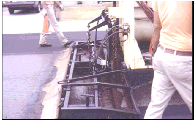
Figure 9- Slurry Seal Box with Augers
