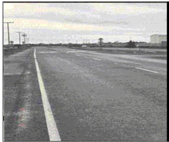
Poor Quality Longitudinal Joints
