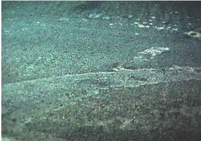
Figure 19- Damage Due to Post Application Heavy Rain with Shear
