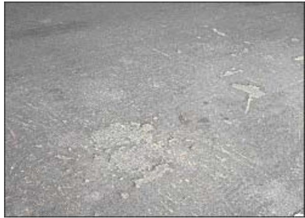
Delamination from a False Slurry
