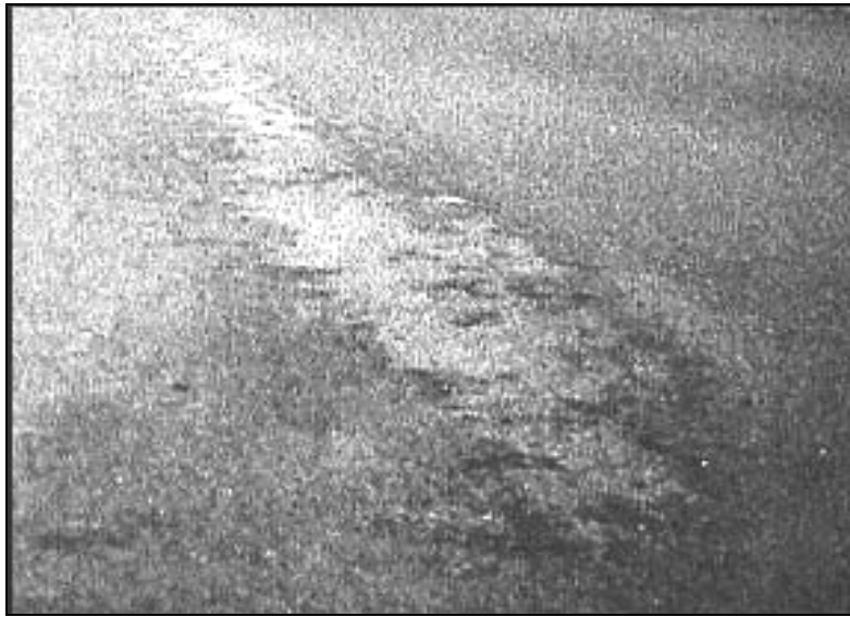
Figure 18-Traffic Damage Caused by Early Trafficking
